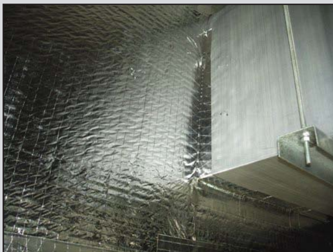
Privacy Board™ sealed at duct penetration
